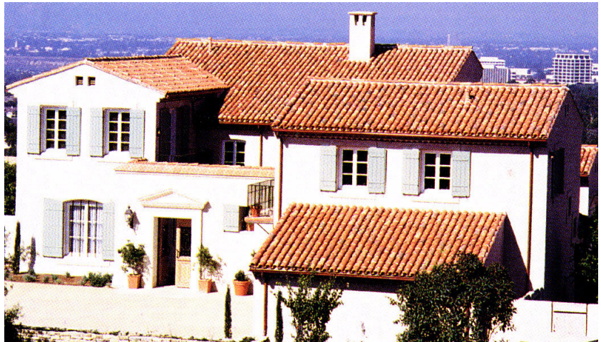
Gable and shed roofs are combined to minimize roof valleys
