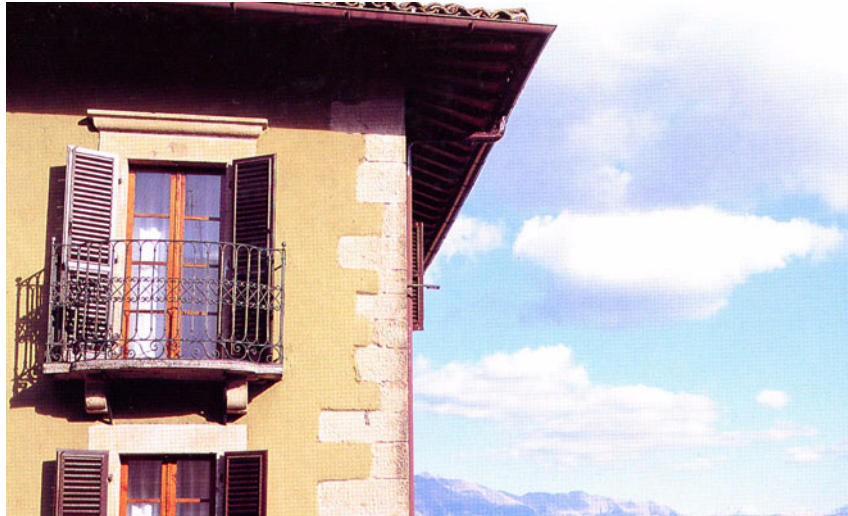
The decorative cast stone balcony is wide to enclose the louvered shutters when in the open position
