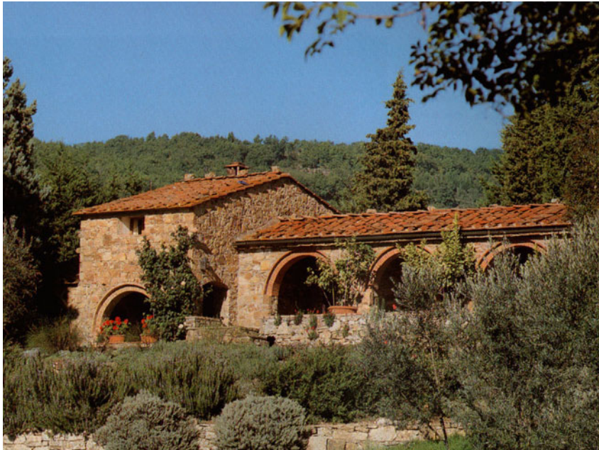
Gable roofs connect at gable walls to avoid roof valleys
