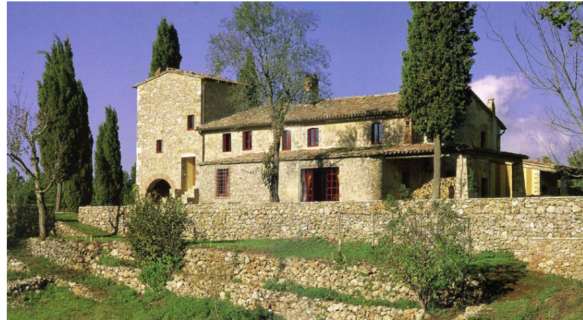
Elevations feature Roman arches, stone with brick framed openings, stacked window alignment and rectangular columns and heavy timber framing
