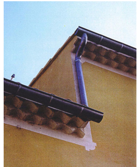
A genoise eave with gutter and downspout
