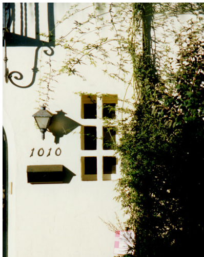
Stucco grilles were slotted brick openings
