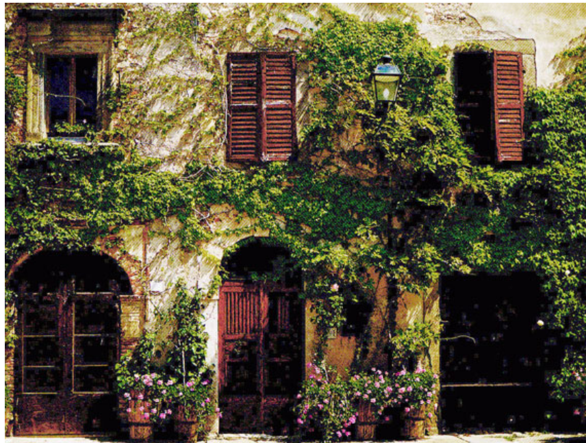
Roman arched openings are reserved for significant rooms. Arched openings should not be stacked over arched openings below
