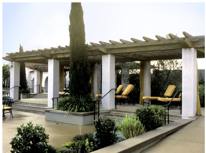
Masonry columns support a well articulated wood trellis
