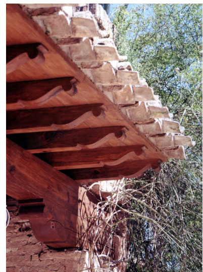
Heavy timber beams support rafter framing with decorative profiles
