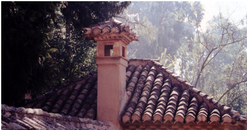
Chimney caps may mimic detailing of the main roof
