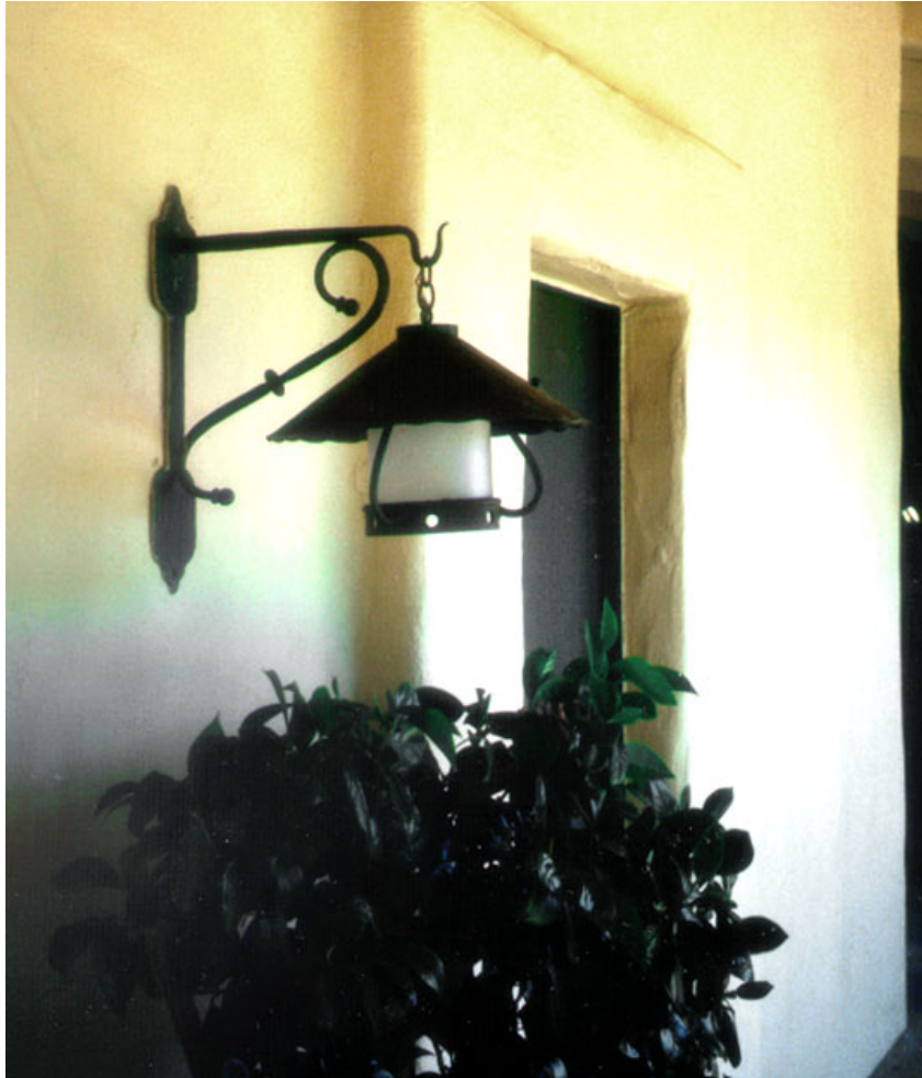
Traditional wall mounted light fixture with light source concealed in hood
