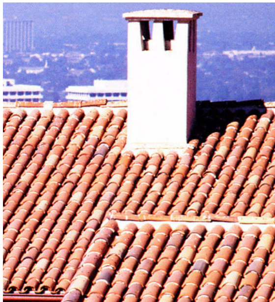
Slightly arched cap terminates this side slotted chimney
