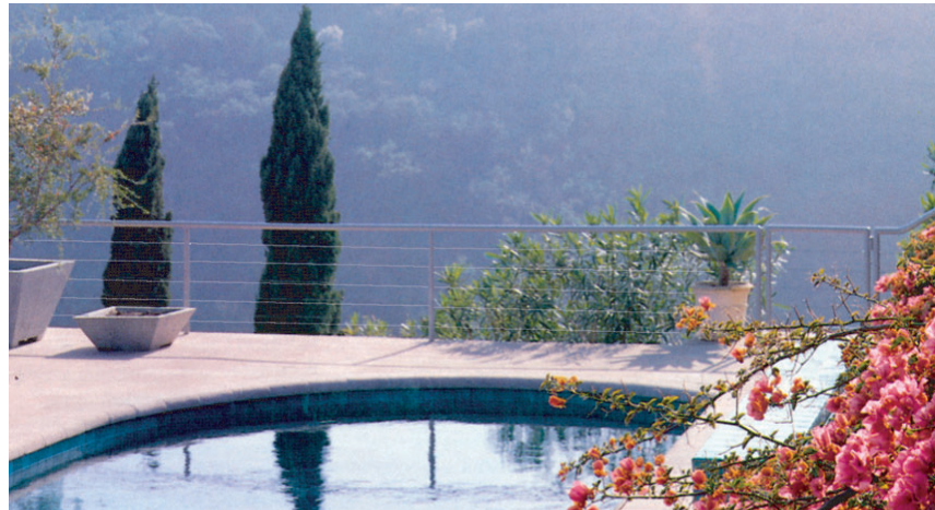
Pool fence constructed with cable that accommodates view
