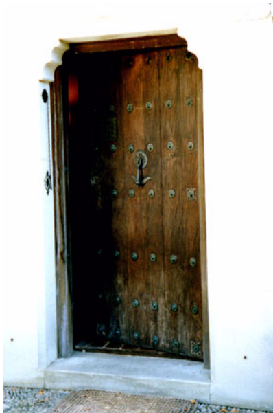
Decorative iron clavos and hand wrought hardware were used to construct entry doors. Door bells are works of art
