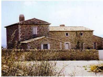
Natural stone walls create a timeless building form. Limestone was used to strengthen building corners and openings
