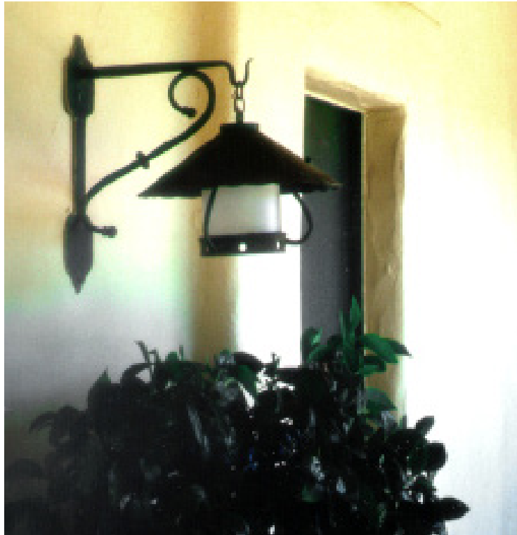
Traditional wall-mounted light fixture with light source concealed in hood
