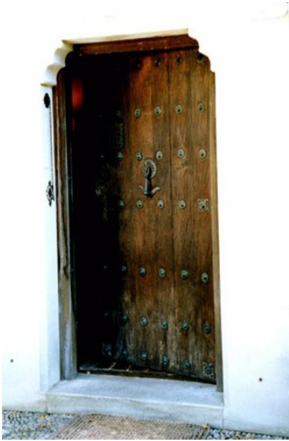
Decorative iron clavoes and hand wrought hardware were used to construct entry doors. Door bells are works of art
