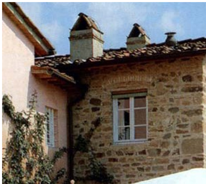
Roof fascias and rakes may simulate plaster corbeled brick
