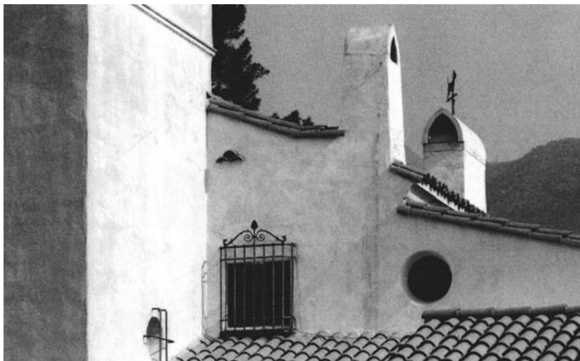
Chimneys were weather protected with stucco finished bonnets or tiled roofs
