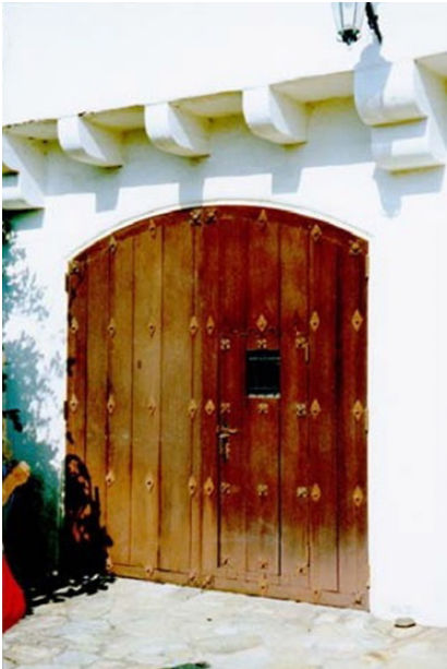
Garage doors employ hinged swing doors rather than overhead closing technology. Speak-easies are common door features
