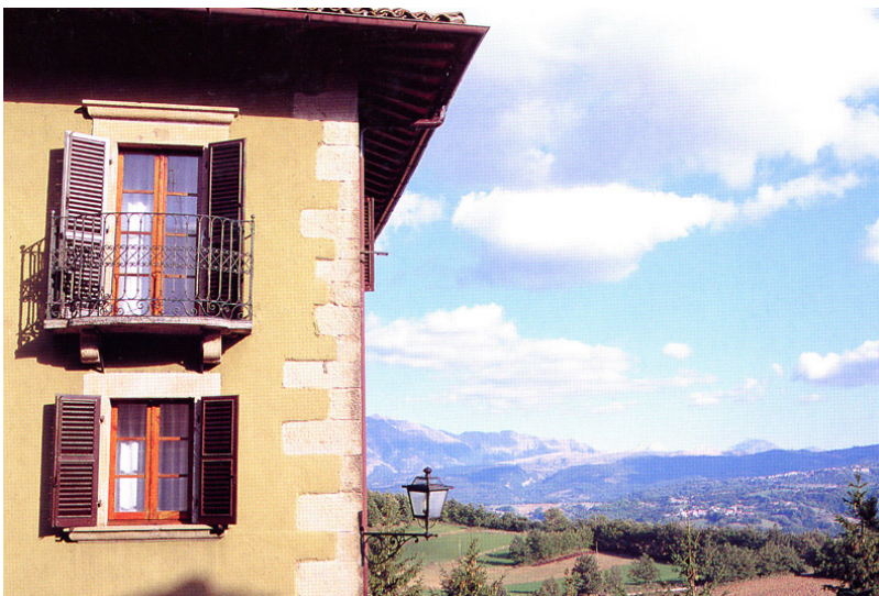
The decorative cast stone balcony is wide to enclose the louvered shutters when in the open position
