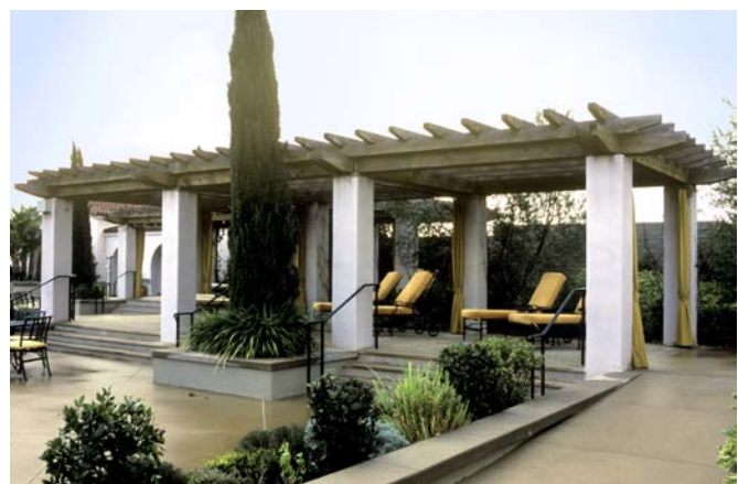
Masonry columns support a well articulated wood trellis
