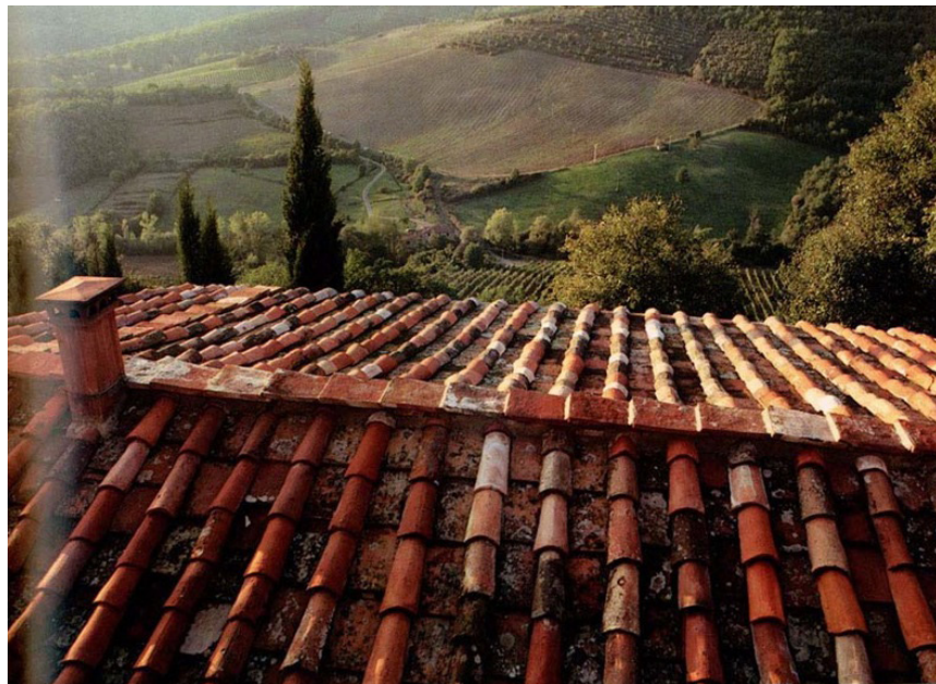
Roman pan clay tile roofs and L-shaped ridge tiles distinguish this roof style
