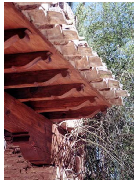
Heavy timber beams support rafter framing with decorative profile
