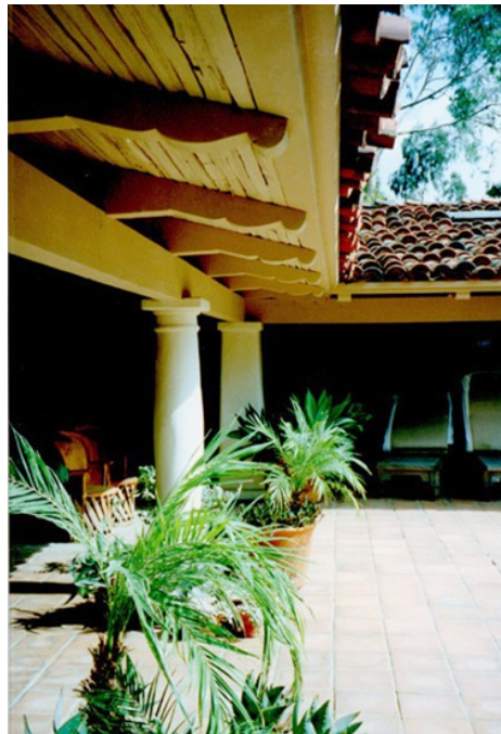
Pre-cast columns and decorative rafter tails add a Mediterranean flavor
