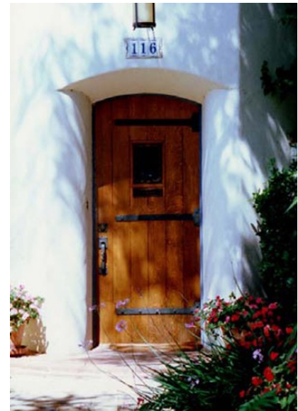
Wood plank door with speak-easy. Radius jambs allow easier opening
