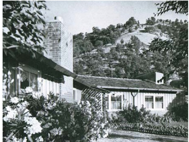
Board and batten wood siding with brick wainscot
