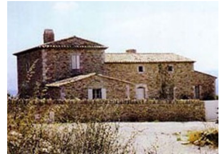
Natural stone walls create a timeless building form. Limestone was used to strengthen building corners and openings
