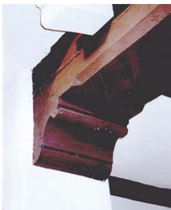
Heavy timber beams and carved wood corbels
