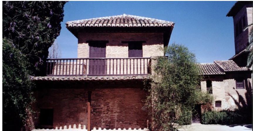
Decorative turned picket, roof tiled edges and heavy timber framing create an elegant deck solution
