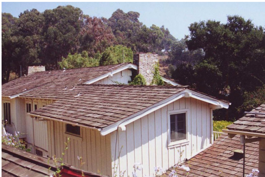
Exposed rafter tails with simplified end cuts
