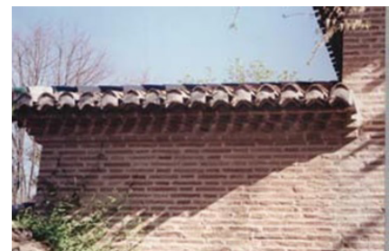
Corbeled bricks support projecting clay tiles with mudded bird stops
