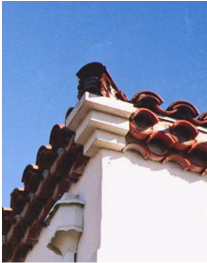
A genoise eave at a hip condition
