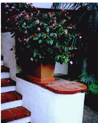
Brick paver treads and brick stepped caps at stair guardrail walls
