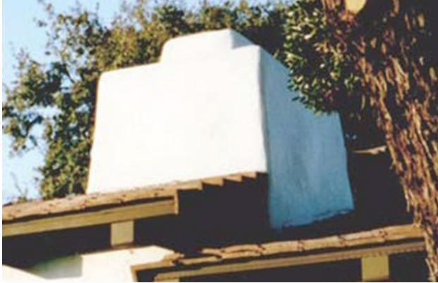
Massive chimneys result from simple and practical adobe construction
