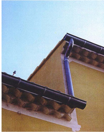
A genoise eave with gutter and down-spout
