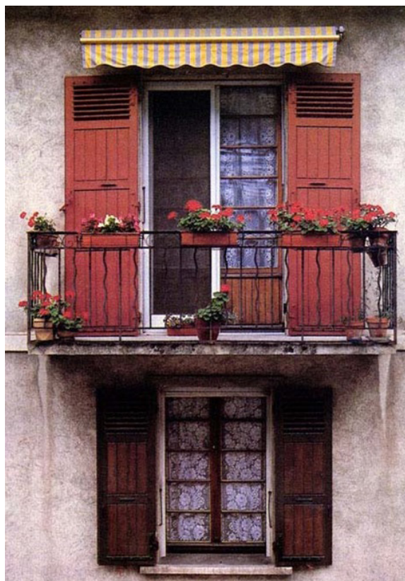
Operable high louvers allowed views outdoors while concealing the observer inside. Wave pattern iron railing pickets area common motif
