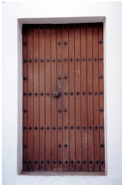
A door knob slightly off center indicates a double swing entry door
